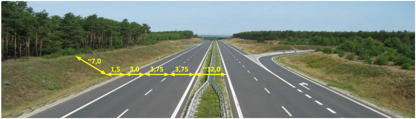
Figure 11. Example of a highway A4 with the following dimensions marked, given in meters: [2 \cdot (\sim 7.0) + 2 \cdot 1.5 + 2 \cdot 3.0 + 4 \cdot 3.75 + (\sim 12.0)] \approx 50.0 [6].
